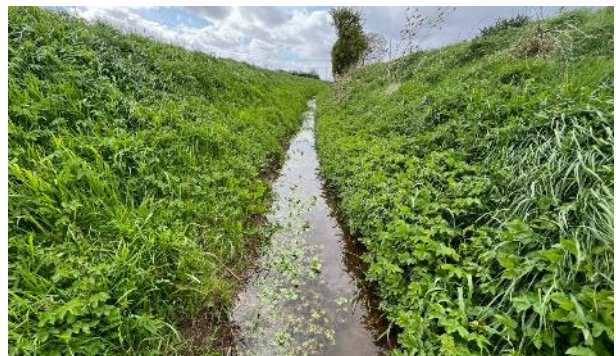
Photograph 7.3.16: Example wet ditch
