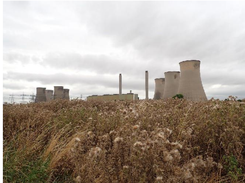
Plate 29 Photograph taken from Scheduled monument, facing north-westwards, towards West Burton power stations
