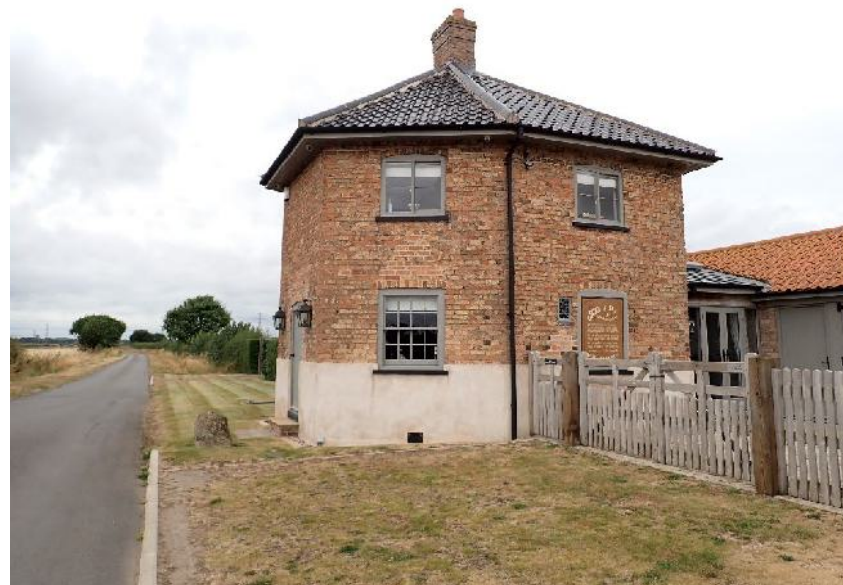
Plate 43 View facing westwards towards Littleborough Cottage
