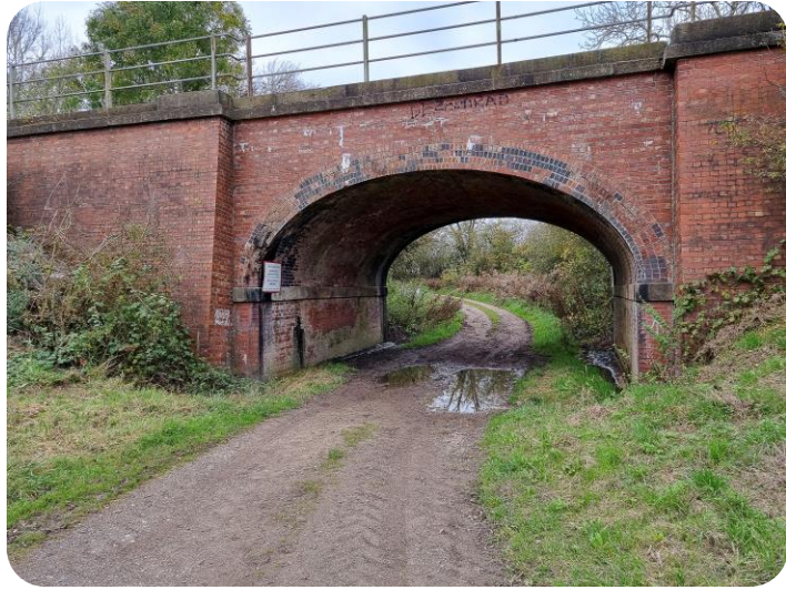
FIG.29 Railway bridge Mac3/207 from Springs Lane
