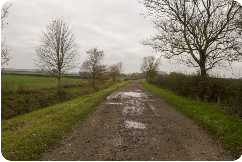
FIG.45 Springs Lane between PV_ARR-11/13
