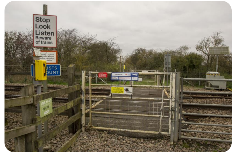
FIG.60 Pedestrian Level Crossing
