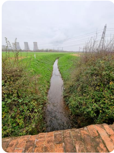
FIG.09 “Catchwater Drain” - view NE
