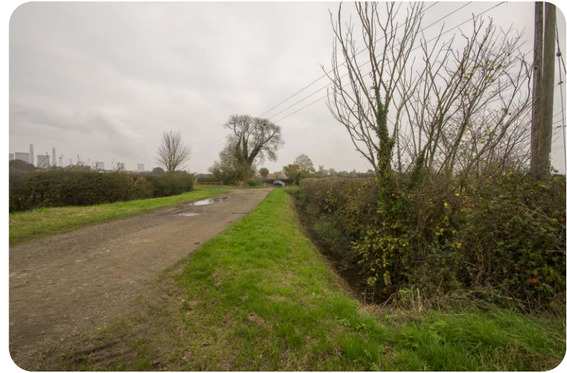
FIG.40 East end of springs lane – drain on right (south)
