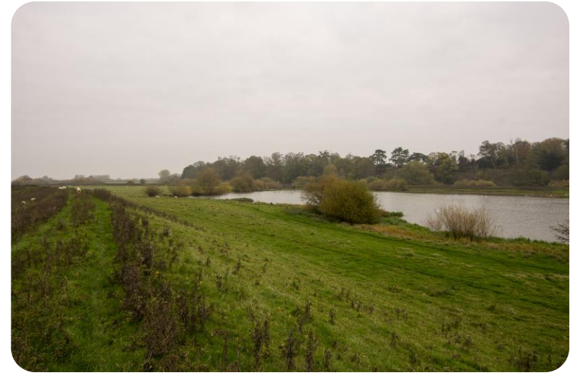
FIG.06 Flood bank and pond
