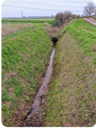
FIG.13 Drainage ditch adjacent Common Lane
