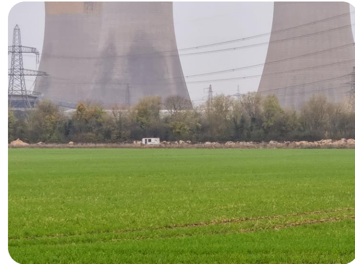
FIG.12 SS_BESS: Road construction, West Burton Power Station
