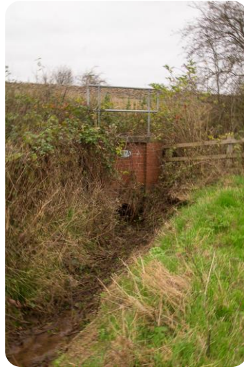
FIG.61 Drainage from culvert under railway embankment
