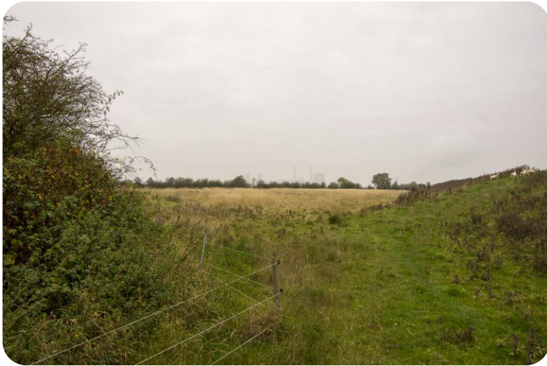
FIG.15 Fields next to flood bank
