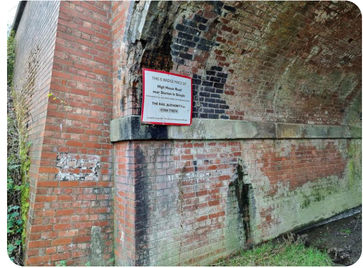
FIG.30 Railway bridge Mac3/207
