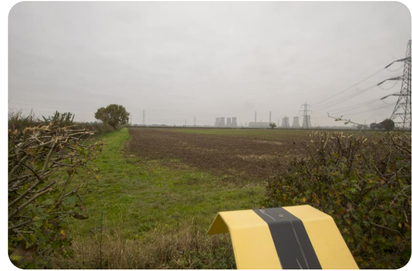
FIG.26 PV_ARR-2 Gas Pipeline marker
