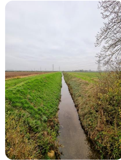
FIG.08 "Catchwater Drain" – View South
