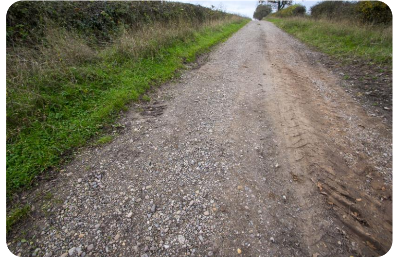
FIG.34 High House Road
