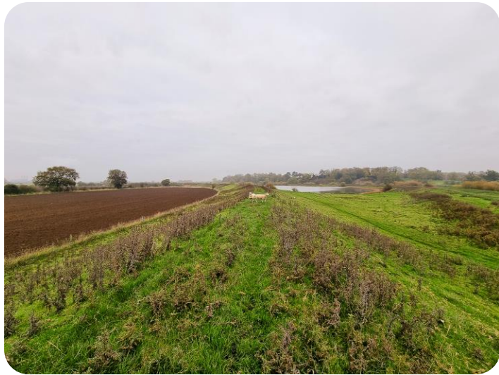
FIG.03 Flood bank crest – view to pond
